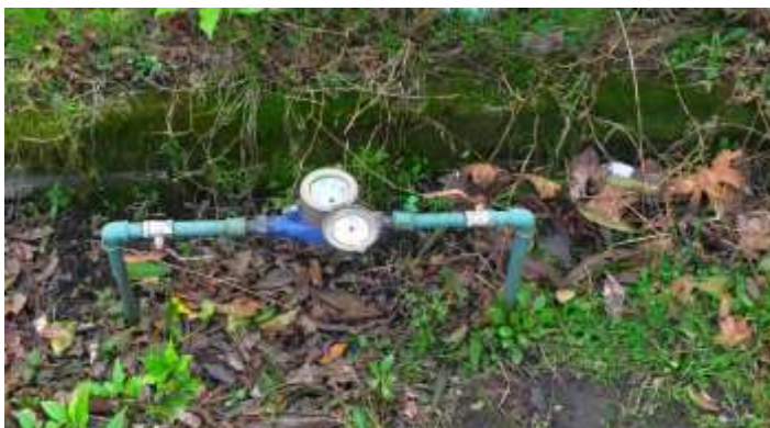
Figure 13 : Airborne water meter installation
