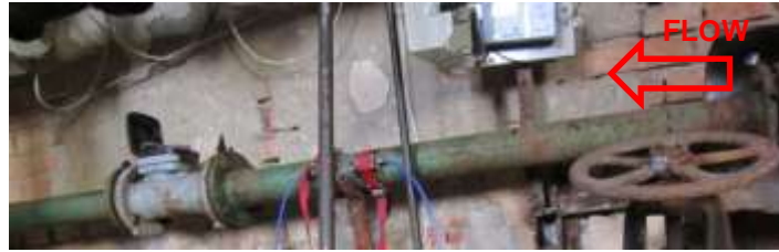
Figure 25 : Metering point configuration before the STVG unit (NON-DOM #5)
