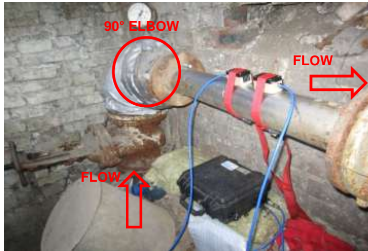
Figure 20 : Metering point configuration before the STVG unit (NON-DOM #2)
