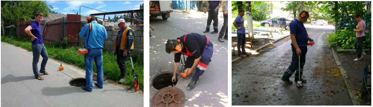
Figure 4: Staff working on ACC water supply network with the provided equipment
