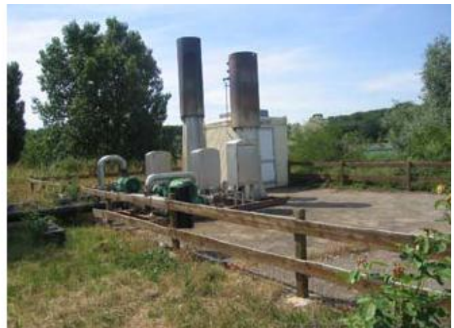
Figure 24 Biogas collection pipes and flaring system at SERAF landfill (France)
