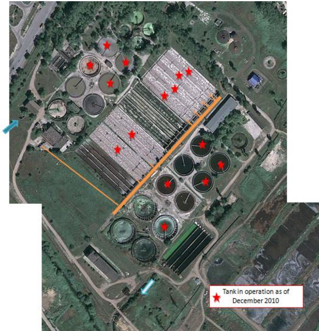
Figure 1: Tanks in operation at Chisinau WWTP
