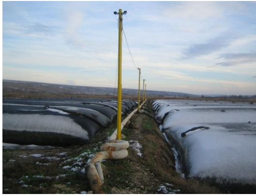
Geotubes with sludge feeding line.
