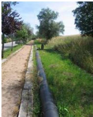
Figure 24 Biogas collection pipes and flaring system at SERAF landfill (France)
