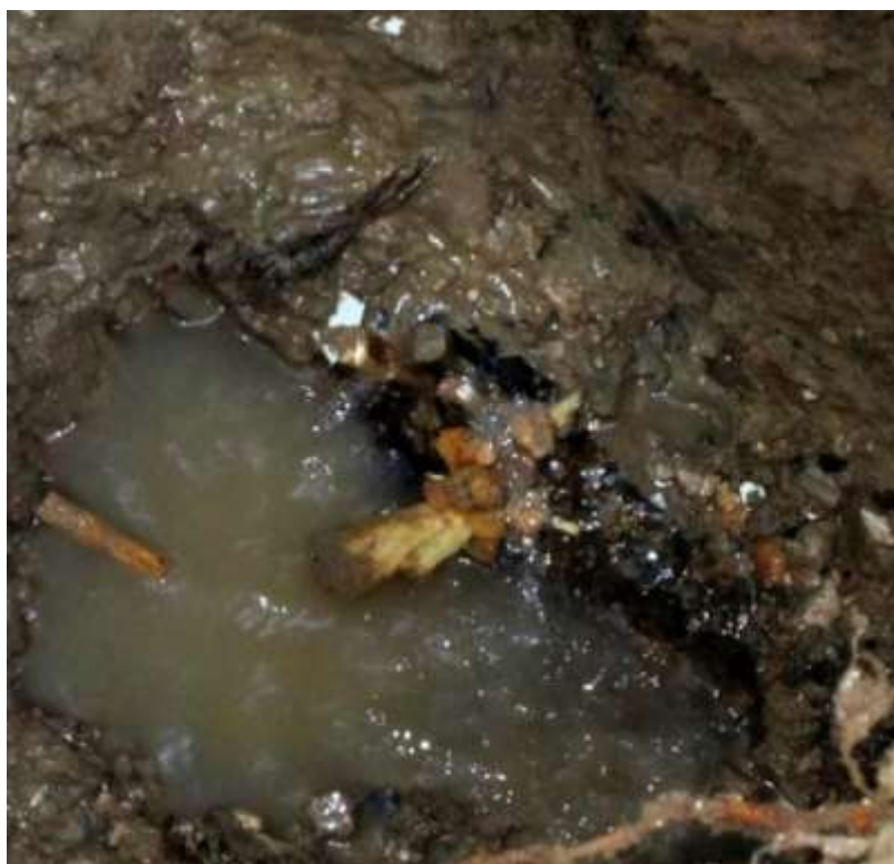
Figure 26: Repair on a pipe using wood cones
