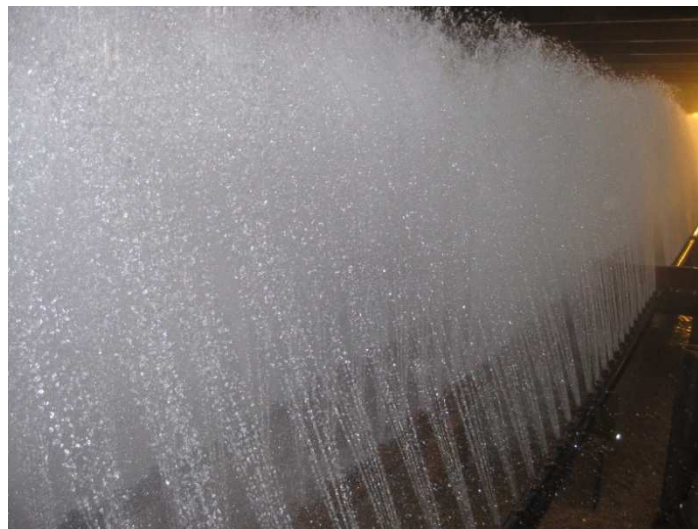
Photo 3: example of aeration with vertical sprinklers
