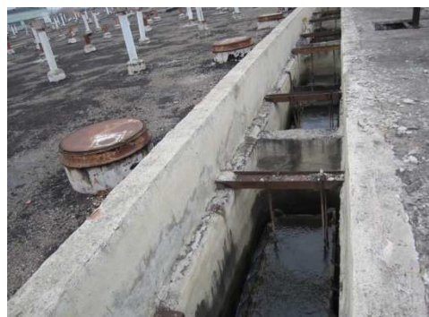
Photo 1: Settlers inlet troughs
