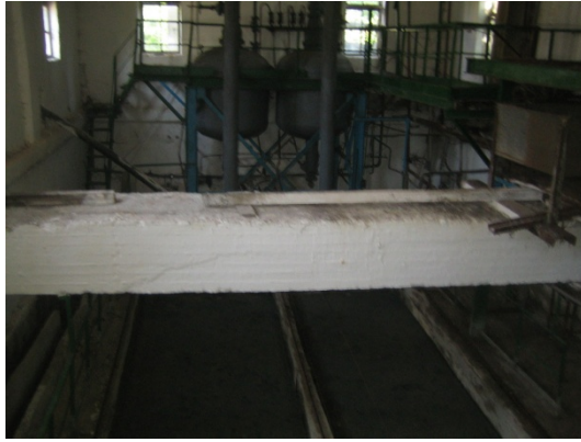
General grease trap with hydrocyclone in the background for grease dewatering
