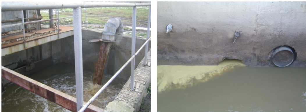
Figure 13: Photos: Second inlet chamber where all influents (industrial and municipal WW) are mixed together with a fraction of the recirculated sludge. The pipe discharges industrial WW. (left) & Inlet of the mixture [leachate from Geotubes + recirculated biological sludge + industrial WW discharged by trucks] at the inlet chamber. (right)
