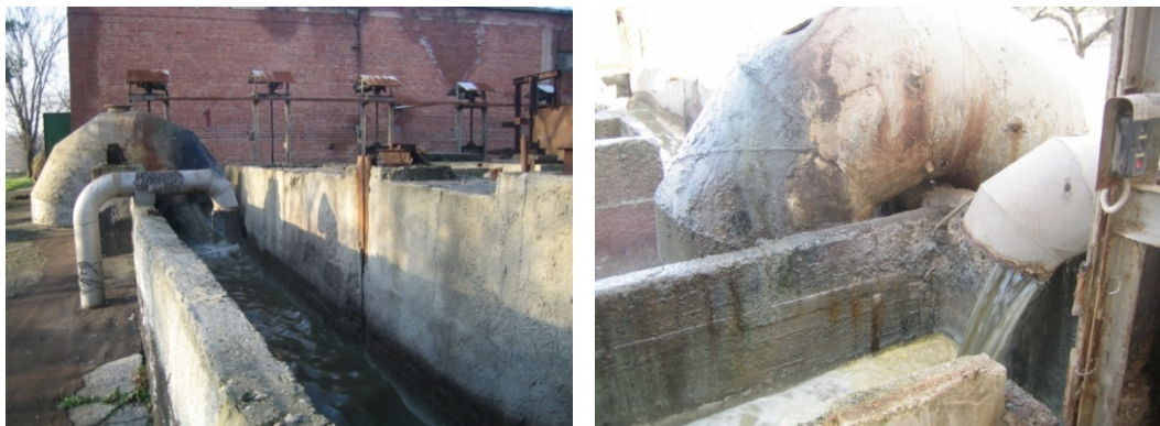
Figure 14: Photos: Open channel which distributes the flow towards the parallel fine screens (inside the building) (left) & Lifting pumps downstream the fine screens (right)
