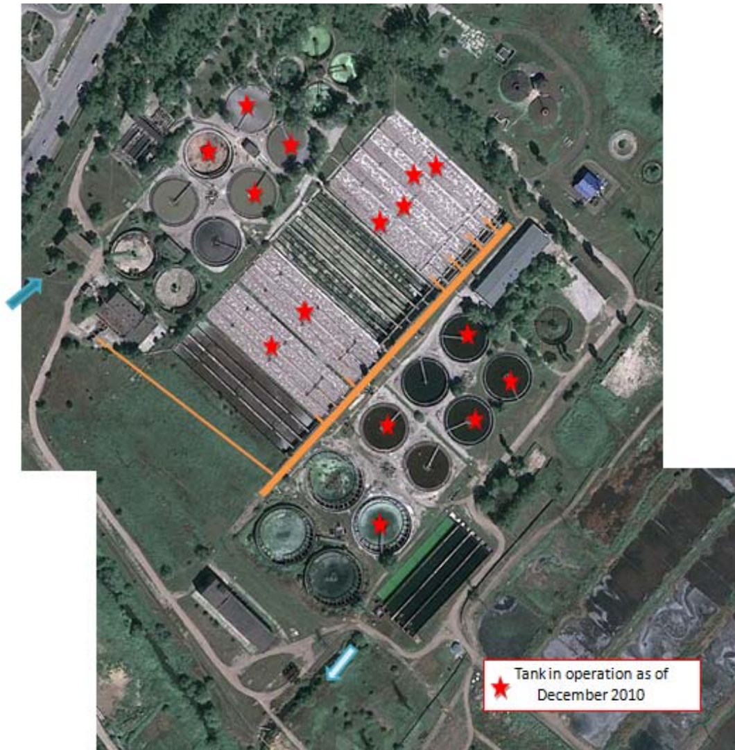
Figure 10: Tanks in operation at Chisinau WWTP
