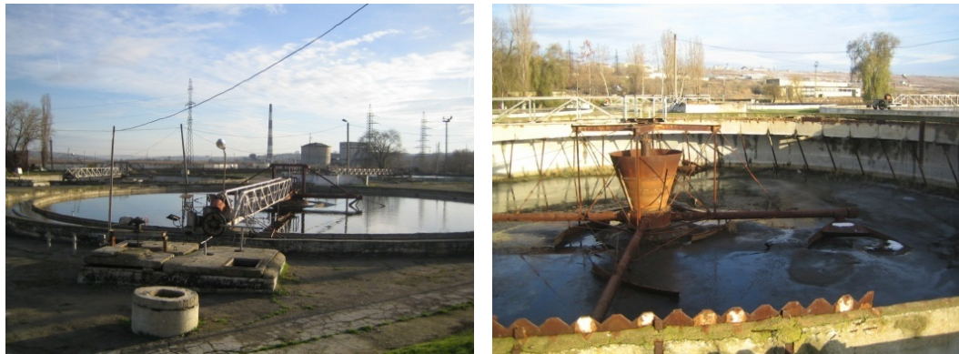
Figure 23: Photos: Secondary clarifier in operation. In the forefront the manually controlled weir that allows the control of sludge withdrawal. (left) & Decommissioned secondary clarifier. (right).
