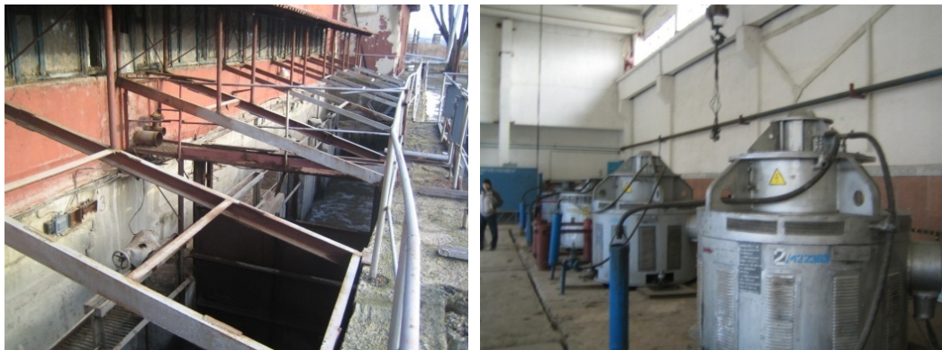
Figure 14: Photos: Open channel which distributes the flow towards the parallel fine screens (inside the building) (left) & Lifting pumps downstream the fine screens (right)
