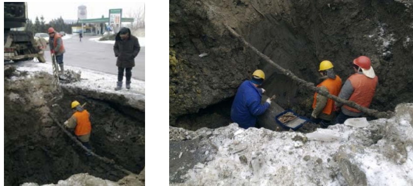
Figure 5-1: ACC DW Sector team at work on a Ø 500 mm
