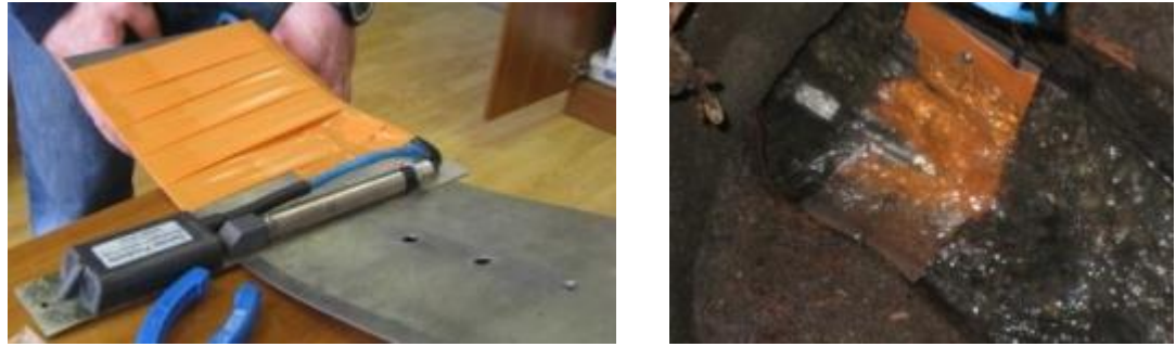
Figure 2.1: Speed and water level sensor – preparation and installation
