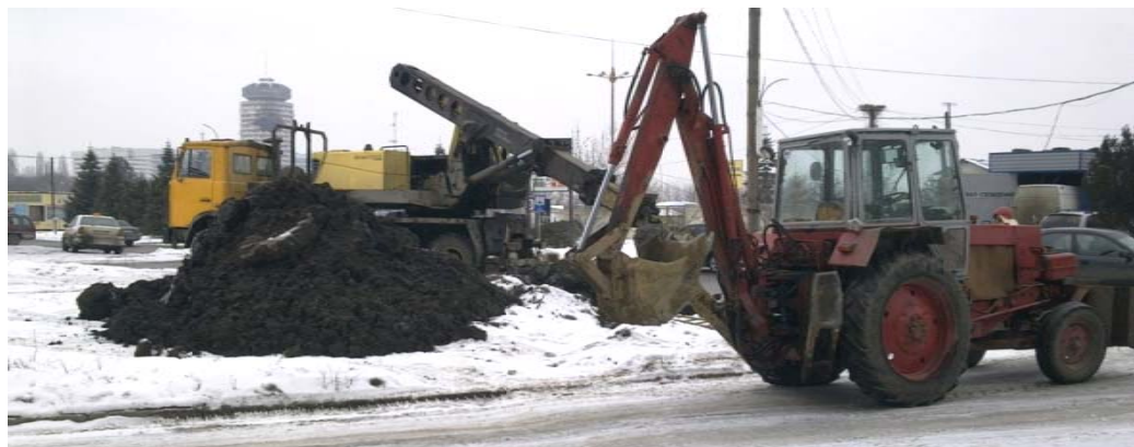
Figure 5-2: Tractor and heavy excavator (from production plant)
