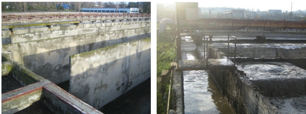
Figure 22: Photos: Decommissioned biological tanks. (left) & Biological tank with the discharge of recirculated sludge in the contact zone (foreground) and the discharge of mixed liquor from the stabilization zone in a common channel (in the background).(right).
