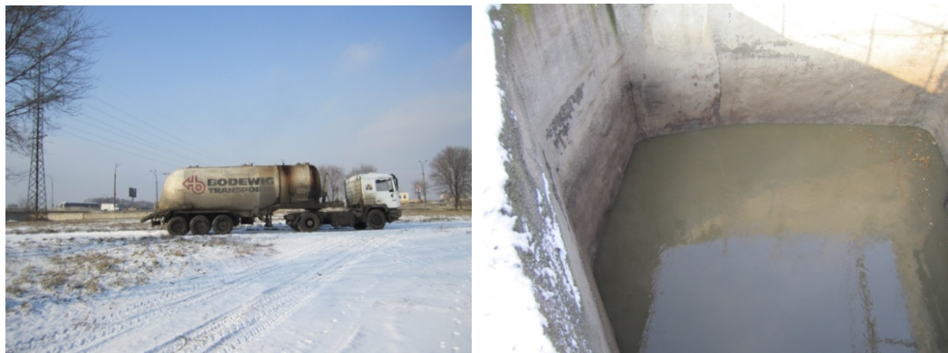
Figure 3: Photos of: Tanker at the WWTP site (left) & First mixing chamber (right)
