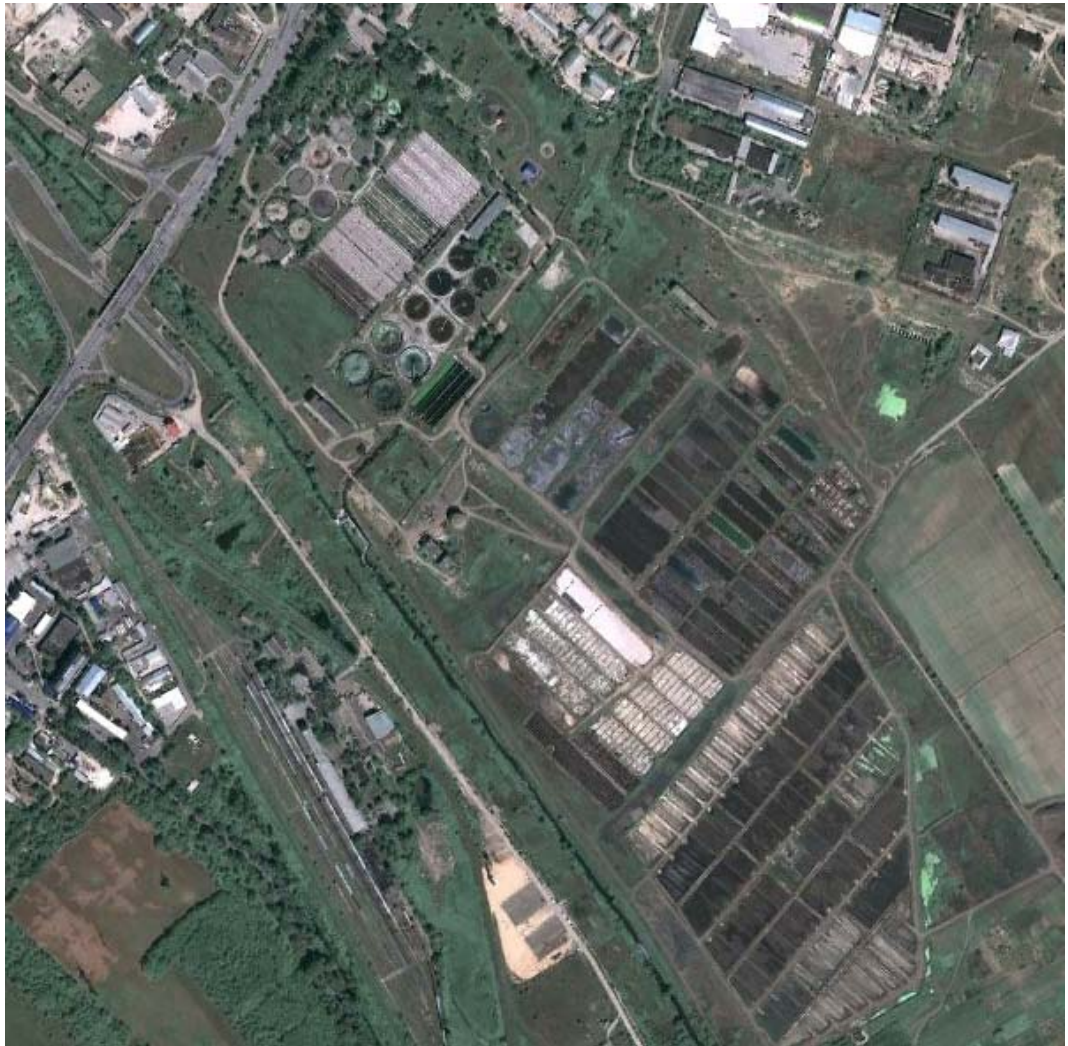
Figure 2: Aerial photography taken on 25/07/2009 of Chisinau WWTP (Source: GoogleEarth, picture taken on 25/07/2009)
