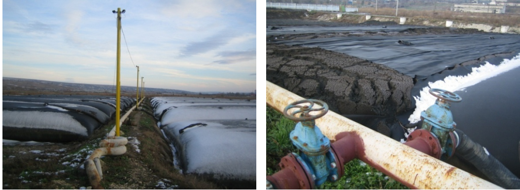
Figure 27: Photos: Geotubes with sludge feeding line.
